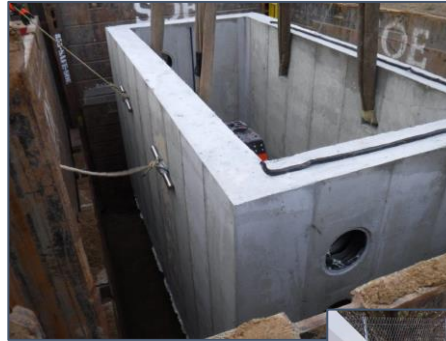
Vault Installation
